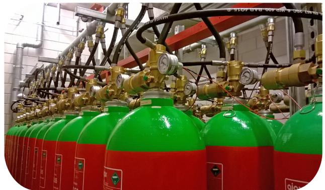
The applied extinguishing gas nozzles are fitted with mufflers. These allow for the minimization of the vibration associated with an extinguishing, thereby preventing damage to data discs.
